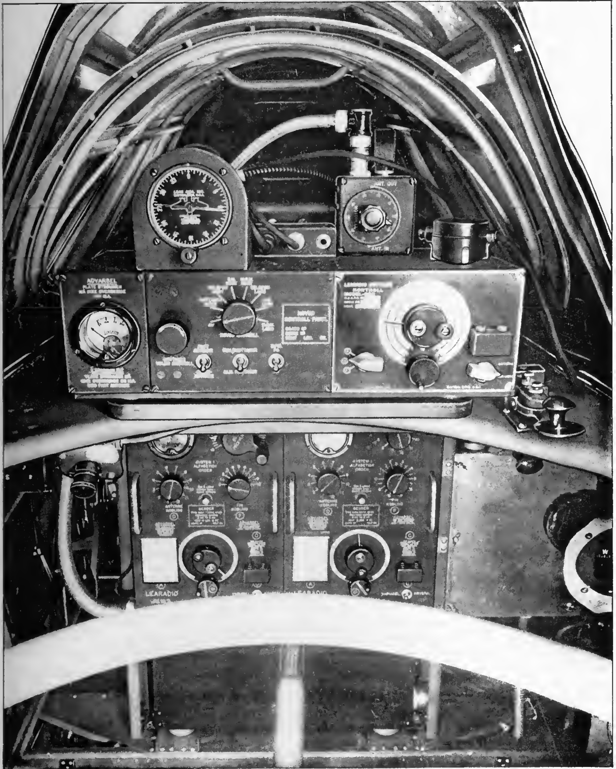
8358 - Radio Installation - Rear Cockpit
